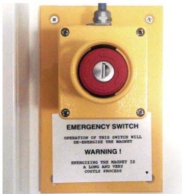
Fig. 2: Magnet Emergency Stop button
